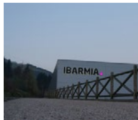
Sun sets over the factory. Each day is an opportunity to keep improving ourselves. That is the philosophy at IBARMIA.
