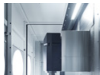
LED lighting in the working area.
